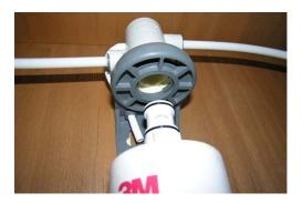
• Install the diverter plug into the filter socket. Insert plug up into the filter socket as far as possible and twist "clockwise" one-quarter turn until it stops.
