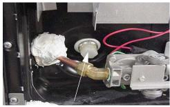
Water Heater Drain Plug (Remove with socket)
