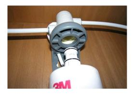
• Install the diverter plug into the filter socket. Insert plug up into the filter socket as far as possible and twist "clockwise" (to the right) one-quarter turn until it stops.
