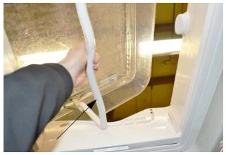
• Pull elevation bar downward to open and raise skylight dome
