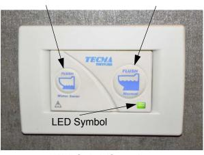
Wall Switch/Controller (Located on wall near toilet)
