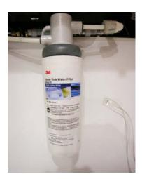
Cold Water Filter Assembly (Located below galley sink) *NOTE: Hot waterline is <u>not filtered.</u>*
