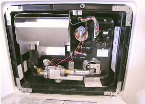
Water Heater Exterior Service Access -Typical View
