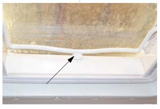
· Press button with thumb to release elevation bar
