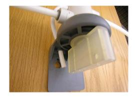
4b. **If Equipped with Culligan Cold Water Filter:** Remove the filter canister from the Cold Water Filtration System under the galley sink and discard the filter cartridge. After emptying the canister, remount it onto the filter assembly and continue the Antifreeze Fill Procedure.
