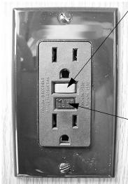
GFCI Outlet (Ground Fault Protector)
